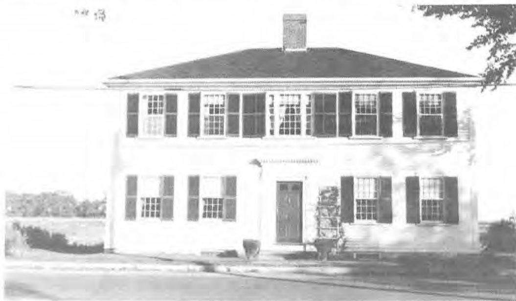
Drew House, headquarters of Duxbury Rural & Historical Society, and location of Soule Kindred office. Picture taken in September 1918 by Donald Walker.
