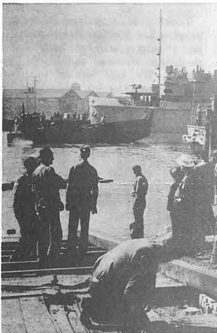
Soulé workers watch another landing craft being launched during the war.
