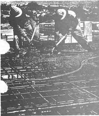
Southern Freeway – San Francisco, California Soulé reinforcing steel
