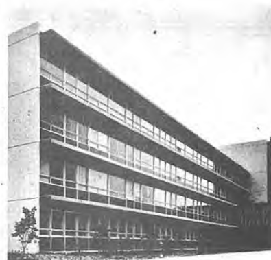
Window wall, attractively designed into this Methodist Hospital project in Los Angeles.
