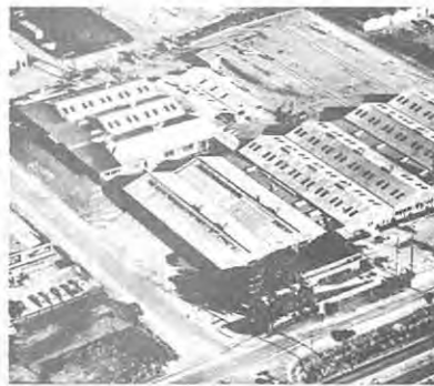
Soulé Buildings (today, we call them Soulé Structures), were introduced by the Company after the War. Pictured here is one of the first major projects, the Lenkurt Electric Company in San Carlos.
