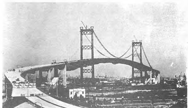
Vincent Thomas Bridge – Terminal Island, California Soulé reinforcing steel
