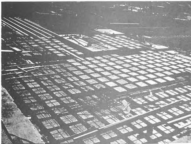
Broadway Hale Store – Los Angeles, California Soulé dome-type steel forms
