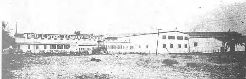
Early scene of Torrance rebar facility. Formerly the American System of Reinforcing, purchase of this Company gave Soule a start in Southern California.
