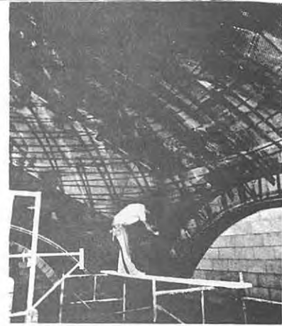
St. Joseph's Monastery – Santa Clara, California Soulé metal lath and channel
