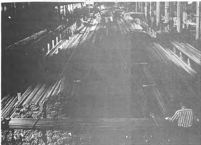
Soulé reinforcing steel warehouse – San Francisco plant
