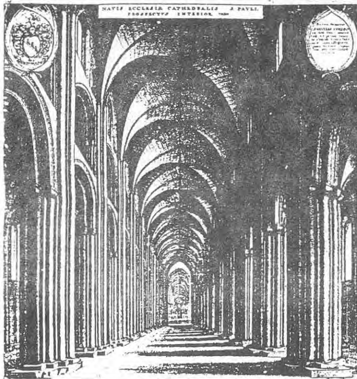
St. Paul's Cathedral, London. The nave, showing the Norman arches and the Gothic windows. The drawing is from a woodcut by W. Dugdale, 1658.
